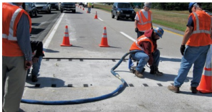
Rys. 2. Wtłaczanie zaczynu cementowego ( http://precast.org/2011/05/precast-concrete-paving-slabs-built-to-last-and-install-fast )
