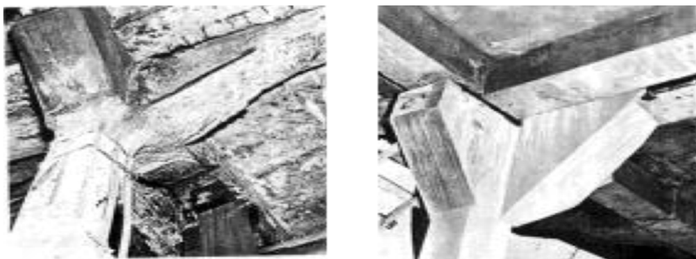
Fig. 1. TSC used in column repair
